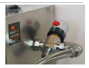
The system will always be shipped with the tempering valve installed.
