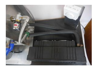
Non-ducted units feature very low power consumption fans that gives their maximum performance when air can flow with minimal restriction. Fan heads should be mounted as close to the area that requires heating as possible. The areas that the fan heads are located must be well ventilated otherwise the fan head performance will be reduced.
