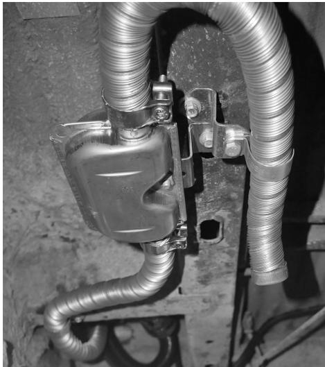
If the exhaust is passing through a timber floor, we strongly recommend using the optional silicon plate, to make sure the exhaust cannot touch the timber, and to ensure there is a water/dust tight seal around the exhaust.
